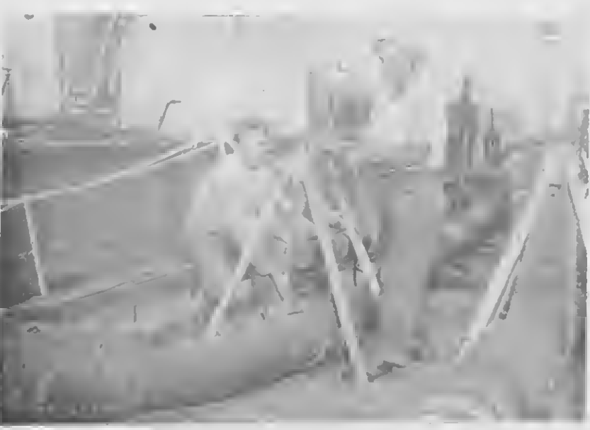
FATHER AND SON: The Receiving and Shipping Department is also proud of its two father and son combinations. The families are the Maduros and the Falconis. Pictured are, left, Arturo, the son, and his father, Benancio. They are shown suspending a 10-inch hose to protect it from damage when pumping action causes it to pulsate.
